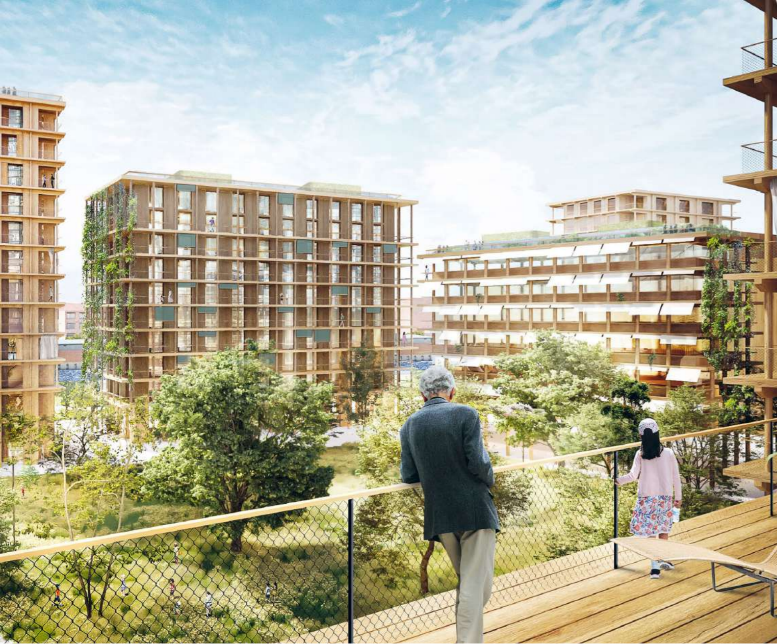
View of the inner courtyard of a residential island (Visualization: moka-studio GbR)
