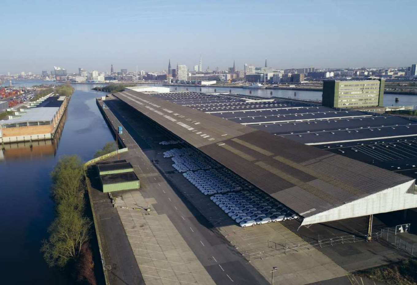
Überseezentrum with its large monopitch roof. In the background, Hafencity and Hamburg city center (Photo: André Dekker)
