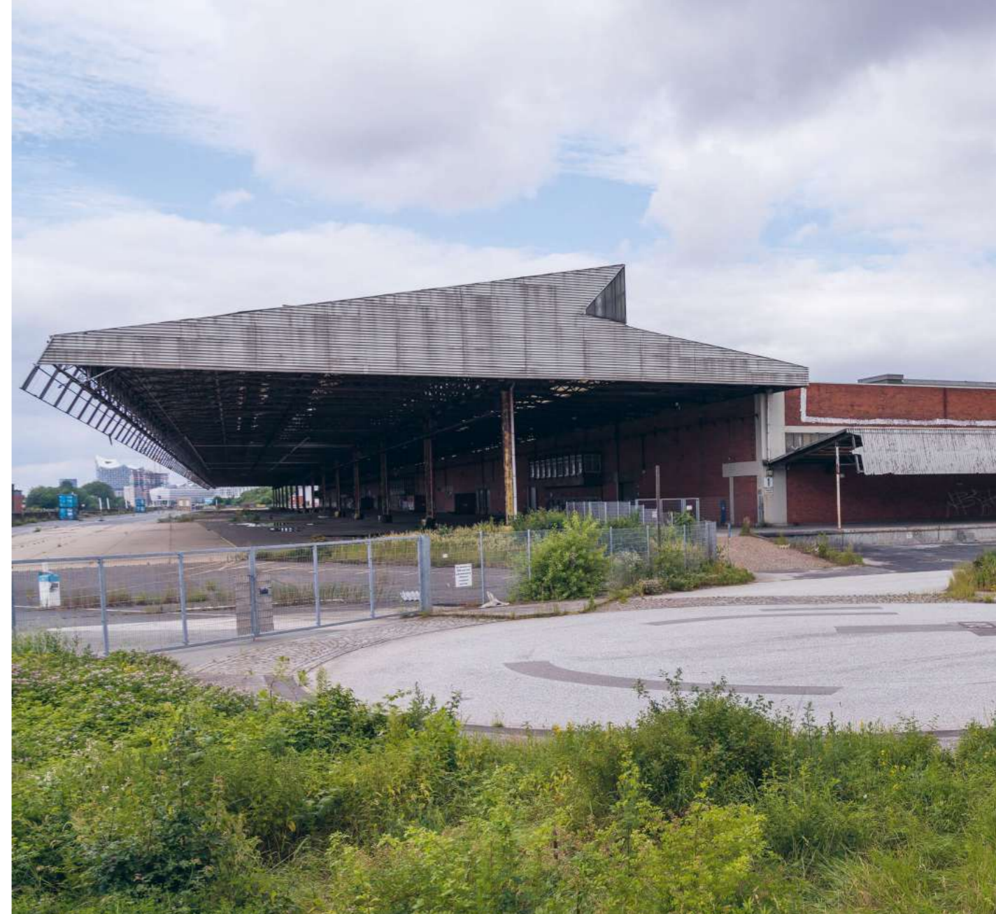
The large monopitch roof of Überseezentrum before demolition (Photo: Thomas Hampel)
