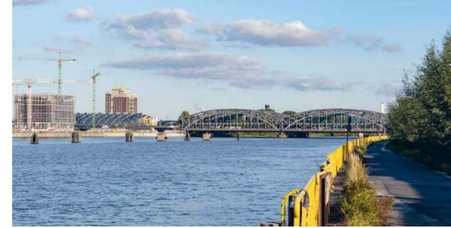
View from Holthusenufer towards the Freihafenbrücke (Photo: Thomas Hampel)
